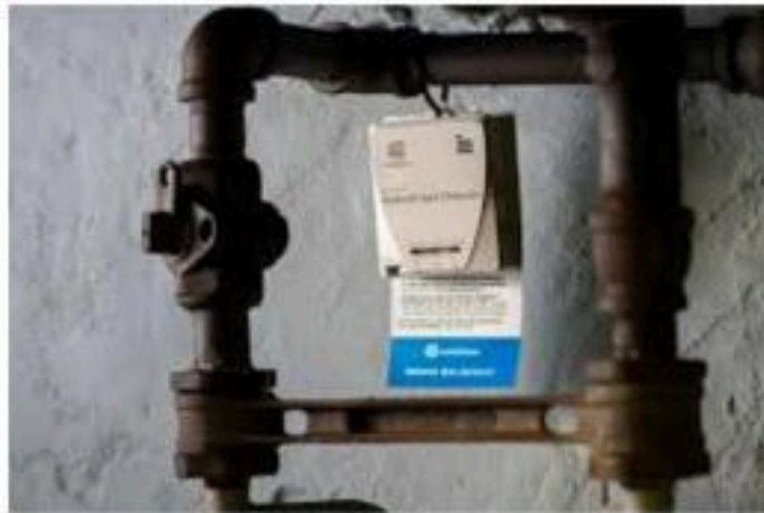
Detectors installed where service enters building
